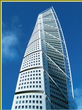
Turning Torso, Malmö-Sweden
