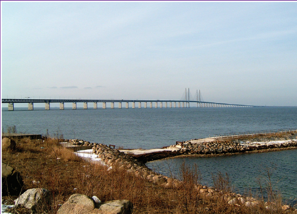
The Öresund bridge, Malmö–Copenhagen
