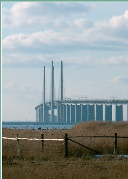
The Öresund bridge, Malmö–Copenhagen
