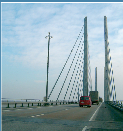
The Öresund bridge, Malmö–Copenhagen
