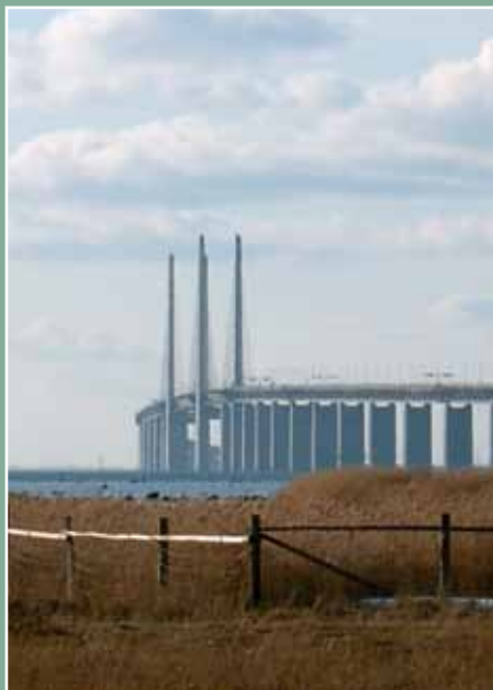
The Öresund bridge, Malmö–Copenhagen
