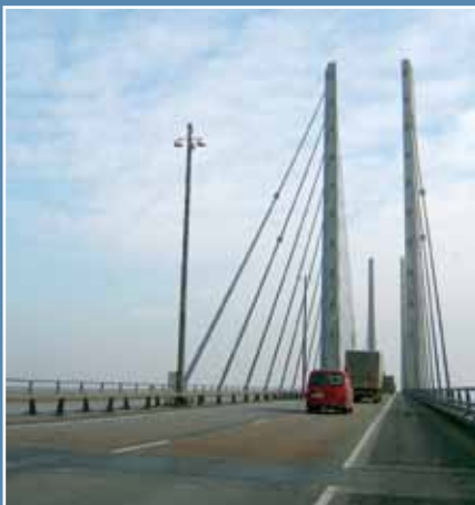
The Öresund bridge, Malmö–Copenhagen
