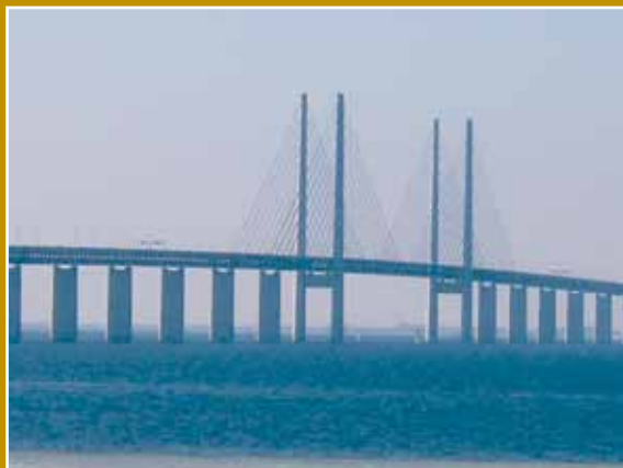
The Öresund bridge, Malmö–Copenhagen
